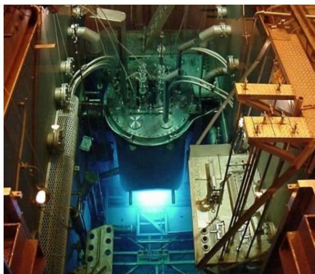
Figure 3 : The SAFARI Materials Test Reactor (MTR) at the Nuclear Energy Corporation of South Africa [18, 19]
