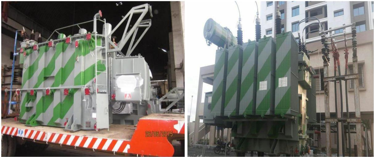
**Figure 3. shows 15 MVA green transformer under dispatch and in service. 15 MVA Green transformer installed at 66 kV Vesu s/s**
