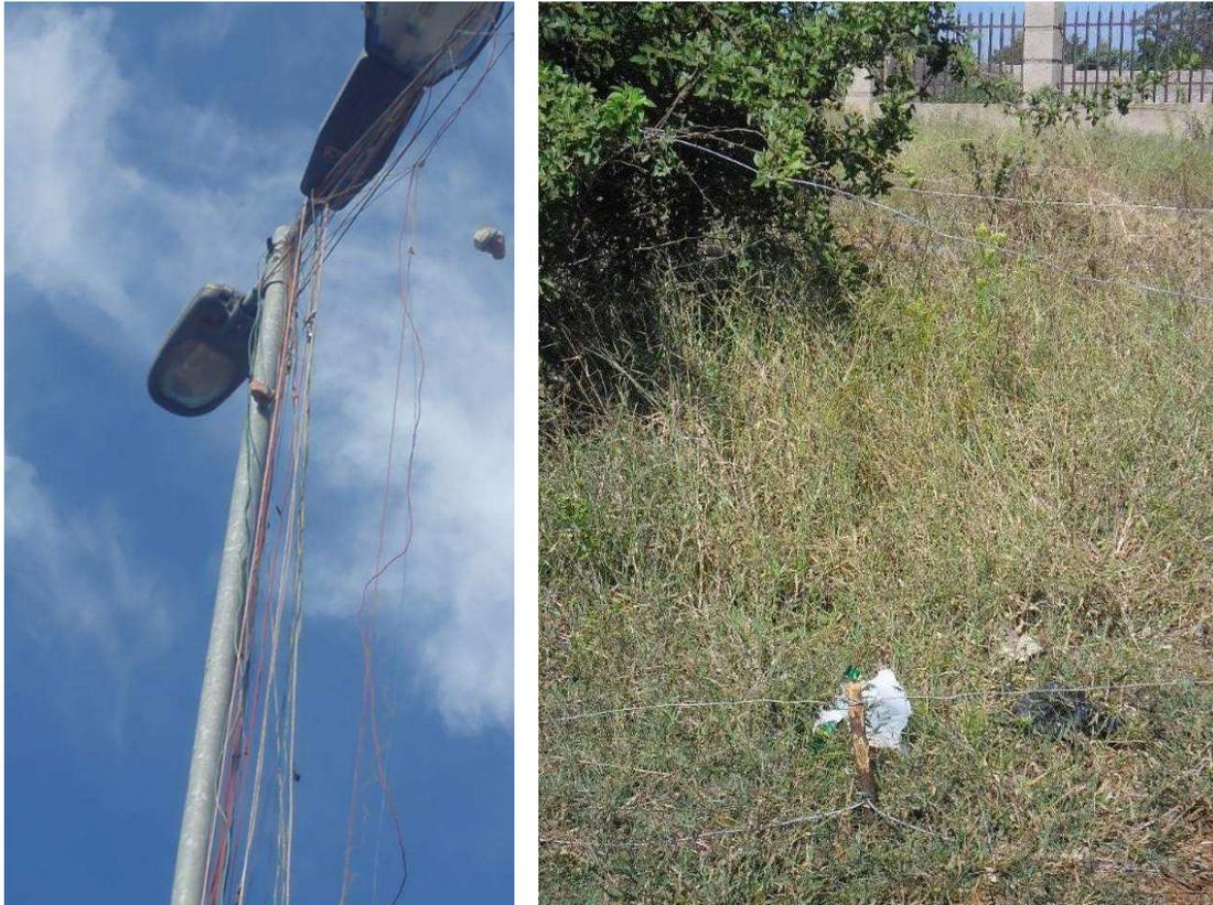
**Fig 2: Examples of illegal connections to a street pole (left) and illegal wires partly concealed in vegetation (right)**
