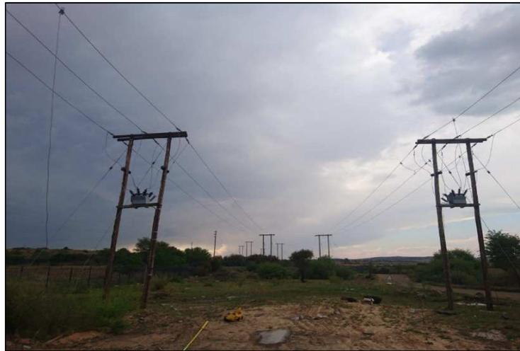
**Figure 3-1 Test site of two 22 kV parallel feeders. An earth fault was created on the line on the left and measurements done on the line on the right**
