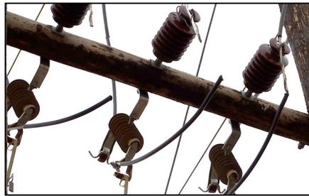
**Figure 1-1 Conductor failures on MV overhead line due to initial temporary fault (lightning) [3]**
