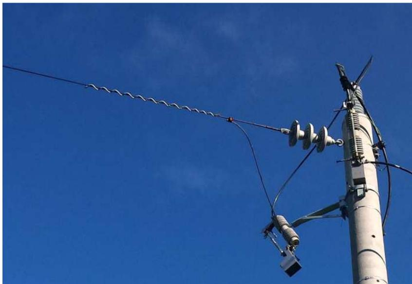
**Figure 6: Covered Carbon Composite Conductor, Compression Dead End, Insulation Piercing Connector (connected to existing downstream electrical infrastructure via insulated 25mm<sup>2</sup> stranded plain hard drawn copper), and Spiral Vibration Damper.**
